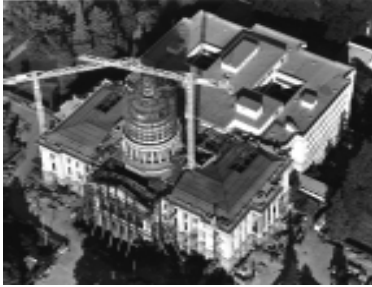
California State Capitol Renovation Complete mechanical renovation ('76)
