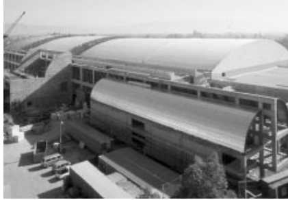
San Jose Convention Center 300' continuous span radius metal roof ('88)
