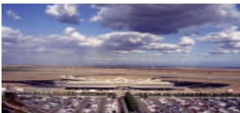
Sacramento International Airport
